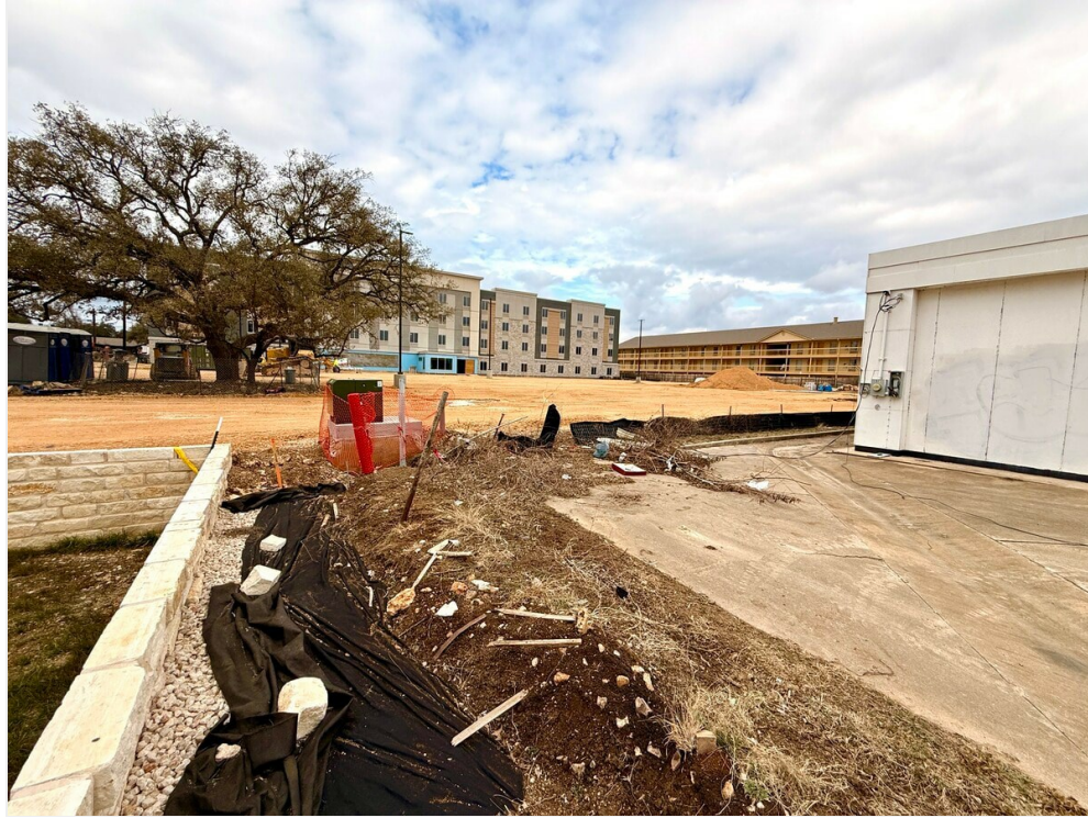
South Side / Hotel construction
