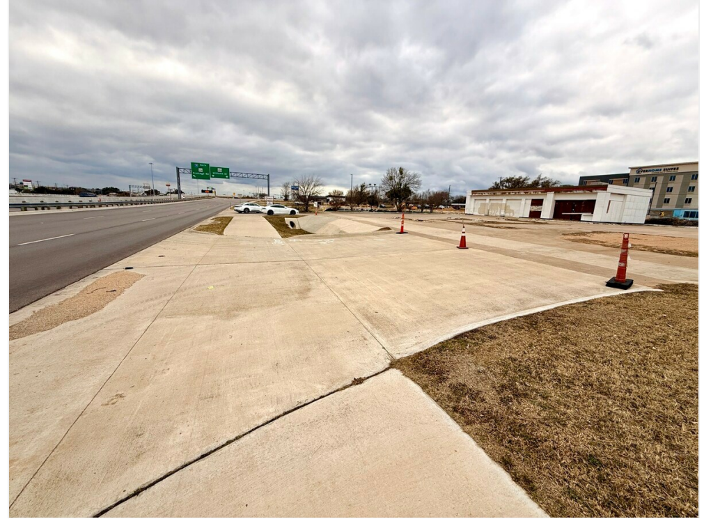
I35 Frontage Road / 2 curb cuts
